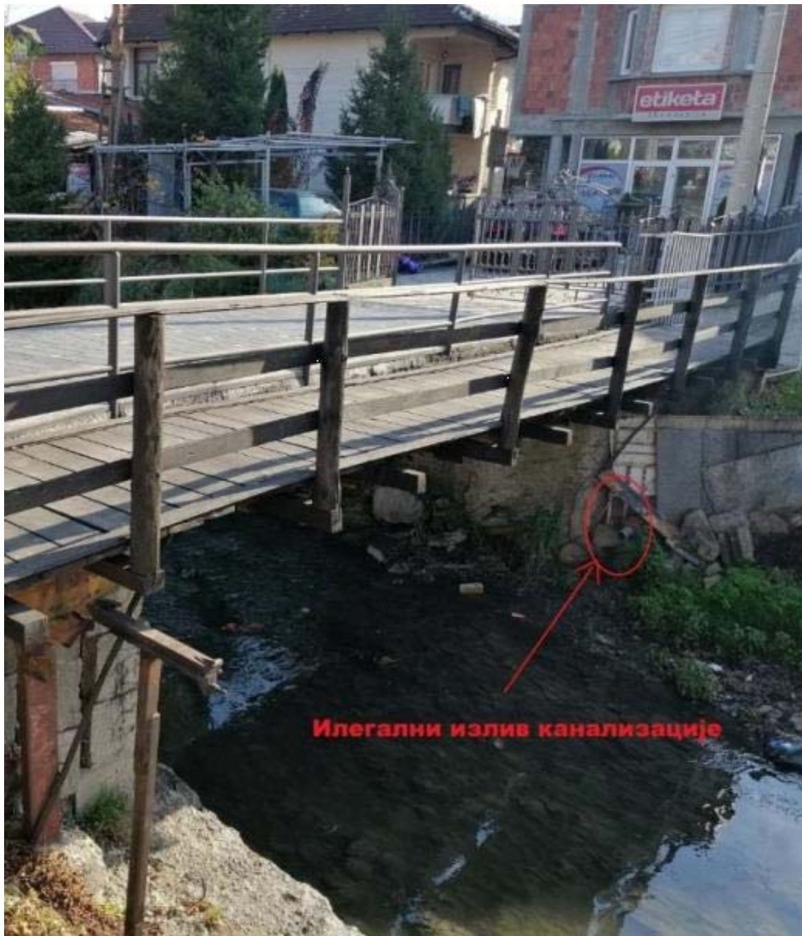
Figure 16: Examples of discharge of sewage directly into a watercourse
