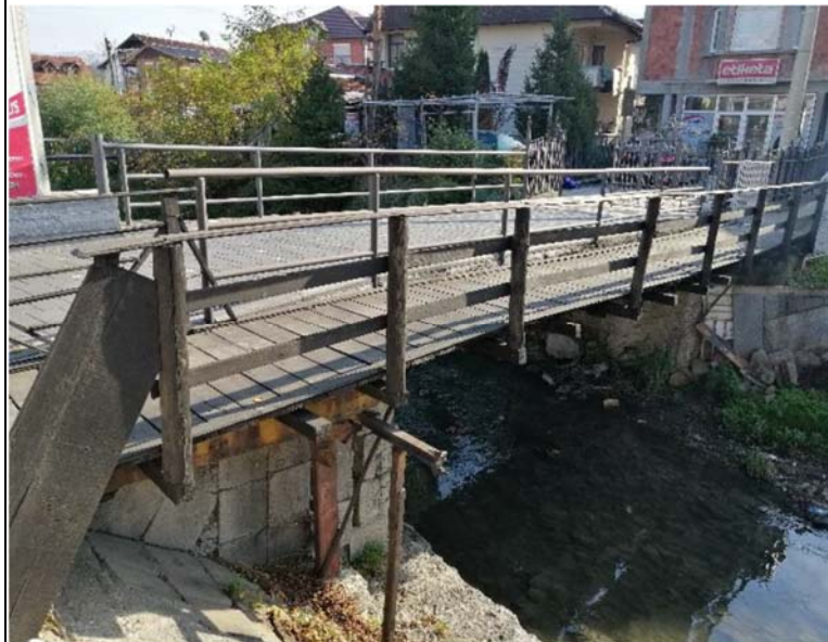
Figure 14: wooden pedestrian bridge on sub-project location
