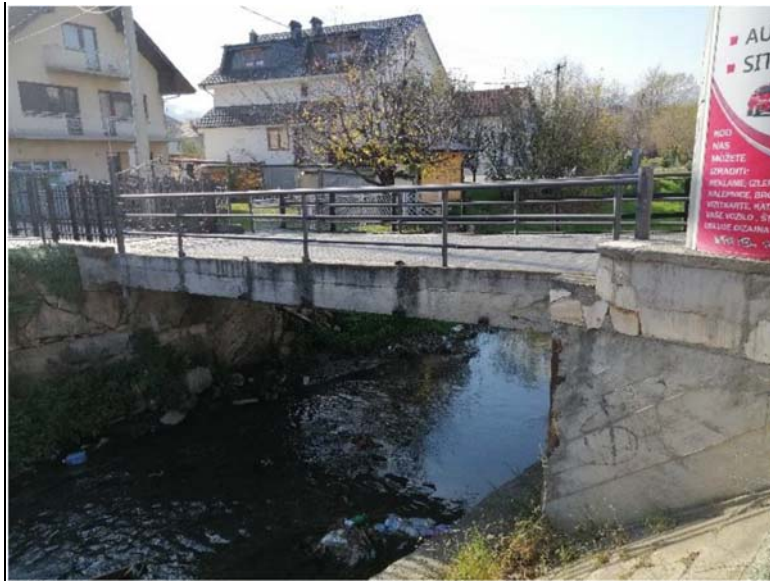
Figure 13: Concrete bridge for vehicles on sub-project location
