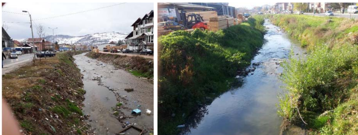
Figure 5: Non trained section of Josanica River through the city of Novi Pazar
