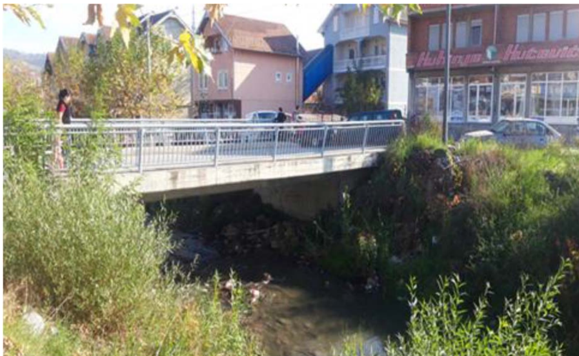
Figure 6: Bridge between trained and non-trained sections (km 0+000)
