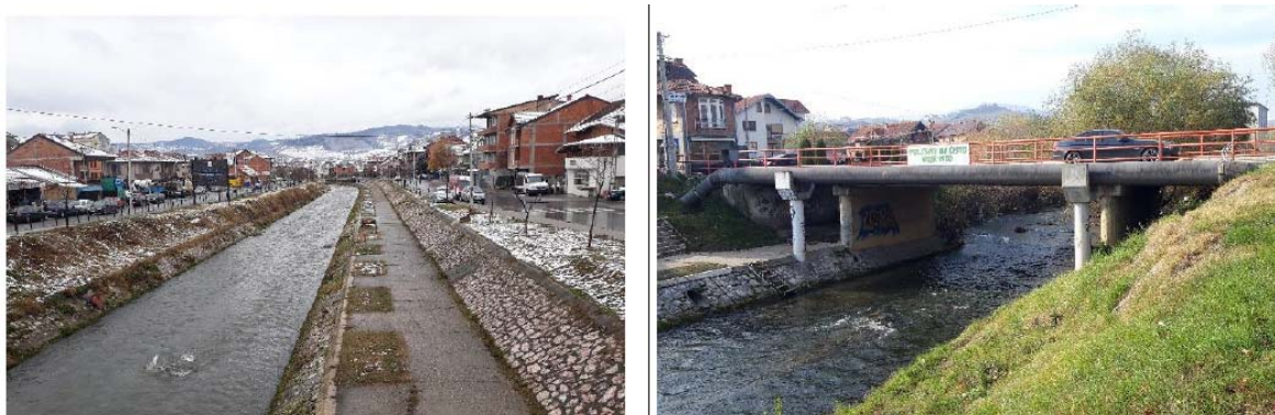
Figure 7: Downstream Training of the Raska River and bridge No. 1 at rkm 0+000
