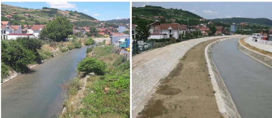
Figure 5: Downstream Raska River training (picture before on the left and after on the right hand side) 2018
