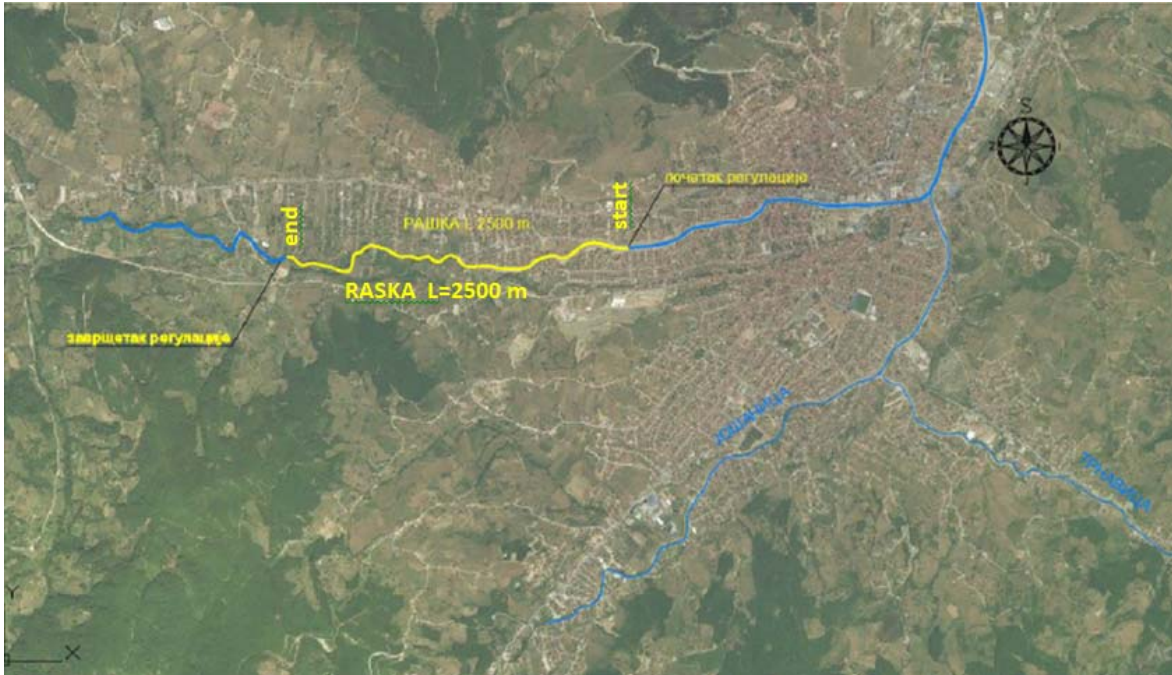
Slika 19: Location of Sub-project section of Raska River in Novi Pazar
